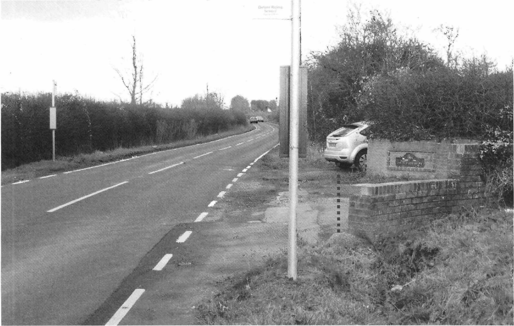
View 1 – showing highway boundary line
